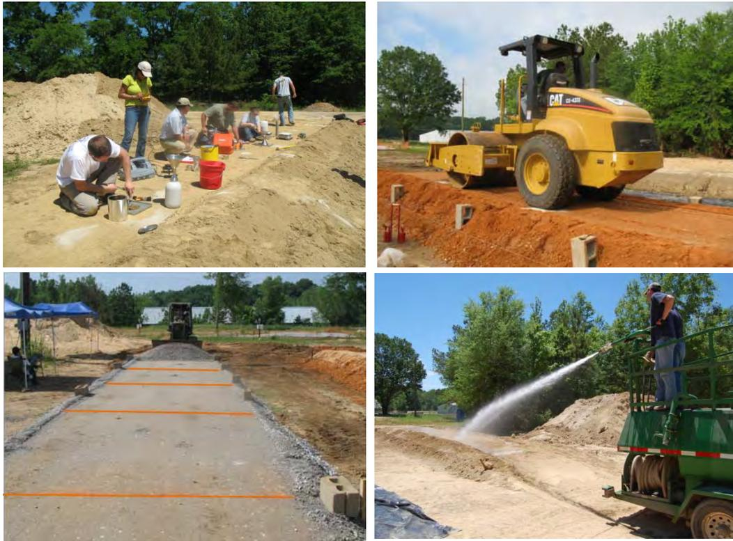
**FIGURE 2 Test Execution. Top left: Device testing on ML-1. Top right: Construction of SP-SC layer (final lift). Bottom left: Construction of GP-GM with test regions marked. Bottom right: Soaking of ML-1 test section following testing of 8<sup>th</sup> coverage.**
